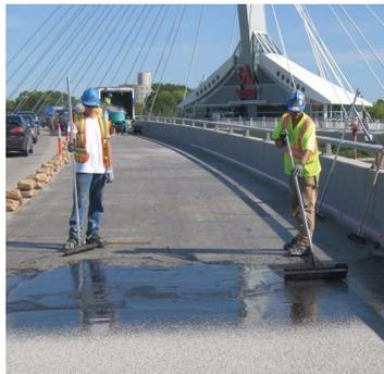
Transpo's T-18 is designed to be applied at 3/8" thickness which eliminates the need to relocate joints, end dams or drain structures. Installation of T-18 will add less than three to four pounds of dead load per square foot of surface area which is an important consideration for rehabilitation of older structures.
