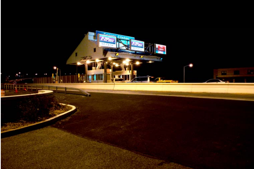
White panels are highly visible on the bridge approach at night
