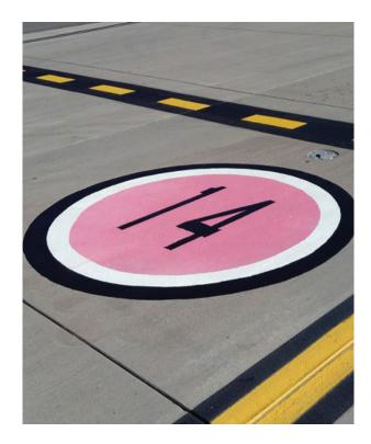
Color-Safe MMA conforms to FAA regulations for taxiway and runway markings: AC 150/5370-10H – Standards for Specifying Construction of Airport.
