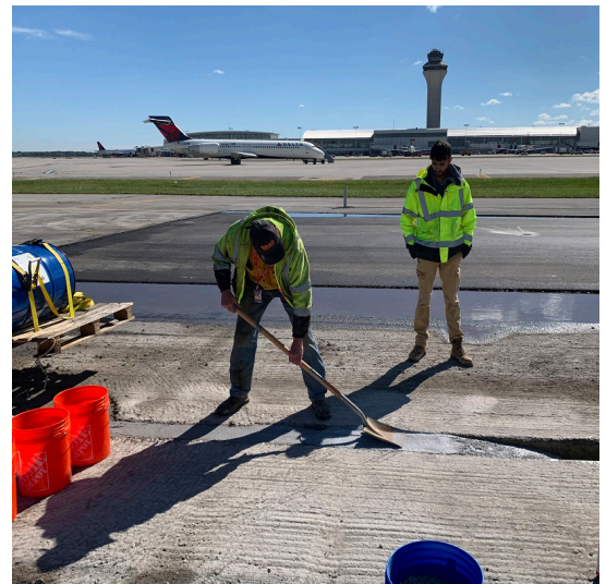
Airport runways repaired quickly with Transpo's T-17 MMA Polymer Concrete Patch Material.
