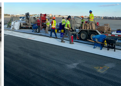
Airport runways repaired quickly with Transpo's T-17 MMA Polymer Concrete Patch Material.
