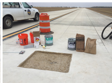
Airport runways repaired quickly with Transpo's T-17 MMA Polymer Concrete Patch Material.
