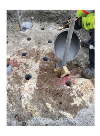
Partial or full depth applications can be accomplished in a single pour, restoring the integrity of deteriorated PCC structures.
