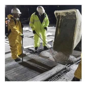
Testing has shown T-17 can be considered an alternative to UHPC
