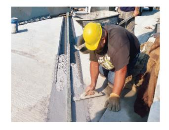
Partial or full depth applications can be accomplished in a single pour, restoring the integrity of deteriorated PCC structures.
