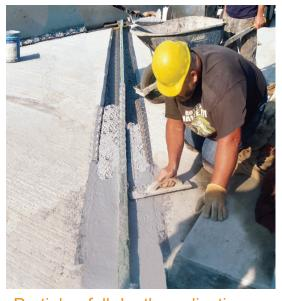
Partial or full depth applications can be accomplished in a single pour restoring the integrity of deteriorated PCC structures.
