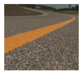
The FHWA has suggested that HFST are the only low cost, active protective solution for roadways, particularly wet or curved surfaces, that is not dependent on driver response.
