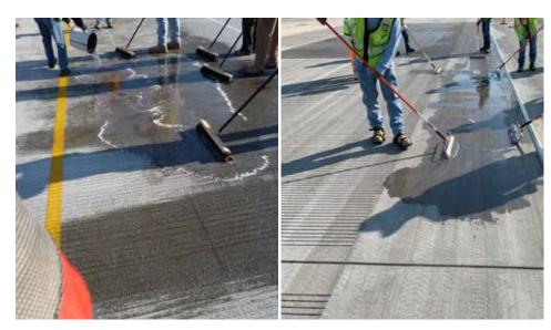
T-78 Polymer Crack Sealer seals cracks effectively and can be open to traffic in as little as an one hour.
