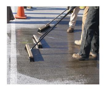
T-78 MMA Polymer Crack Sealer seals cracks effectively and can be open to traffic in as little as an one hour.
