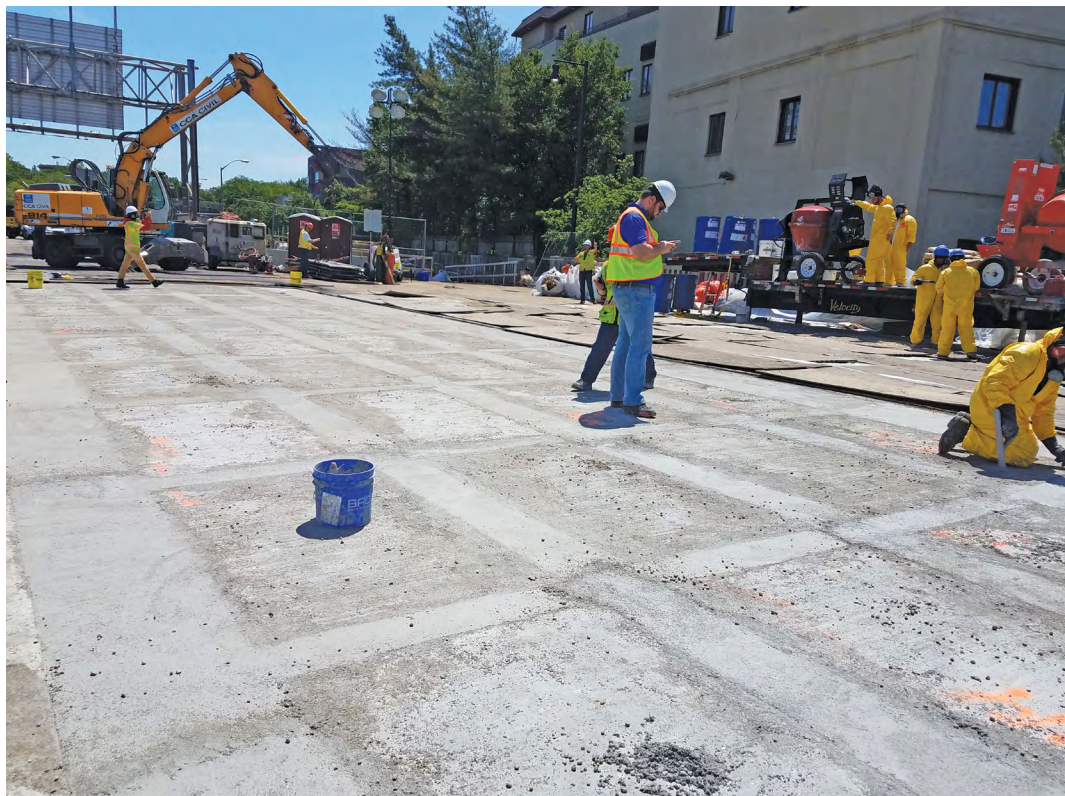
Polymer concrete is made of organic hydrocarbons that act like superglue, giving it high bond strength and durability. It won't corrode with salt and can be used for repairs.
